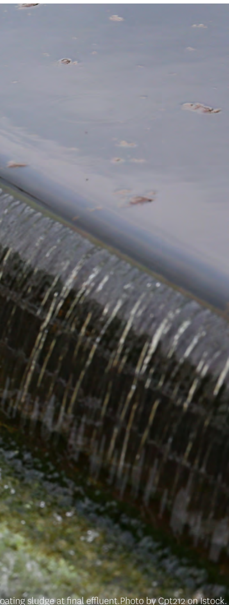
oating sludge at final effluent. Photo by Cpt212 on Istock.
