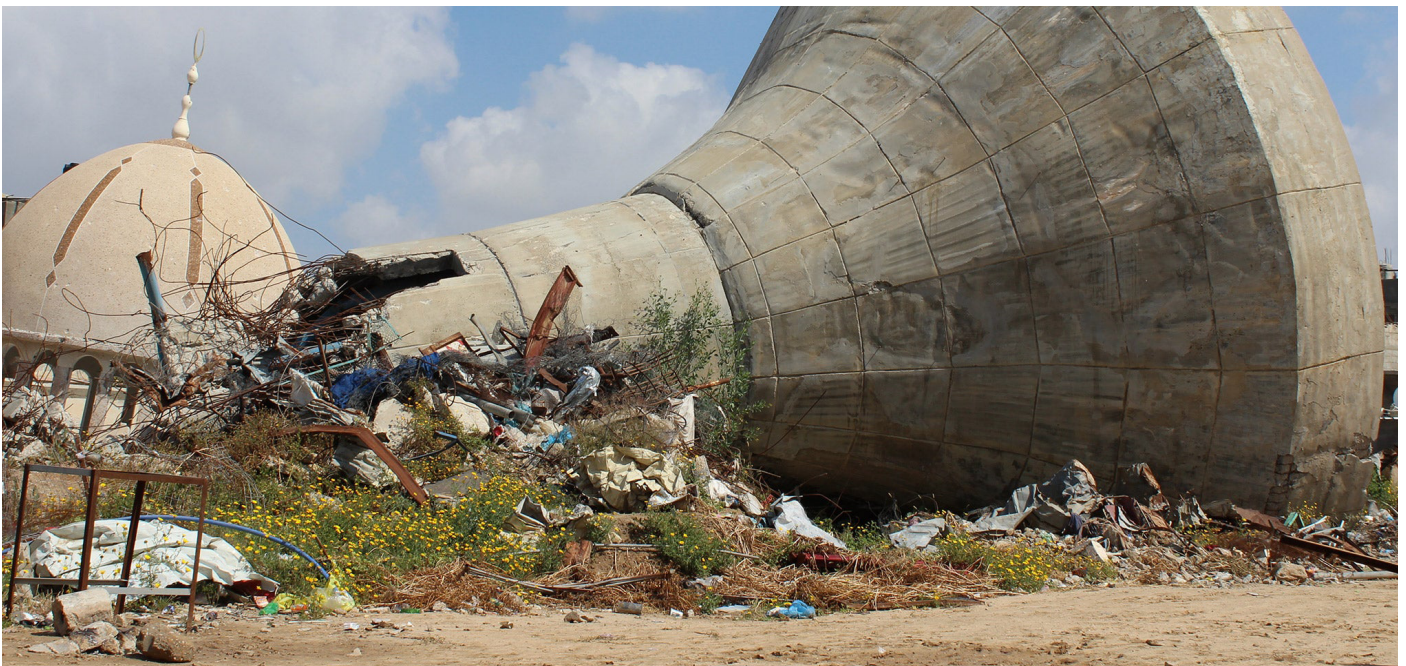
Water Tower destroyed in Khan Younis, Gaza 2014. © CAFOD
