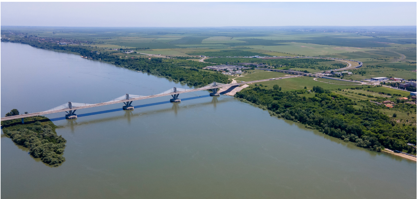
The Vidin-Calafat Danube Bridge provides a reliable link between Bulgaria and Romania. © Stoyan Haytov
