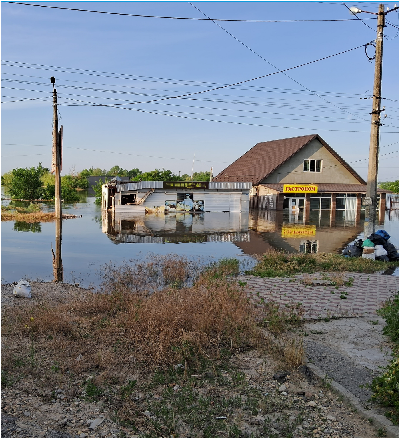
Flooded building after the destruction of the Kakhovka dam, Kherson region, Ukraine 6 June 2023. © A_sm on Adobe Stock
