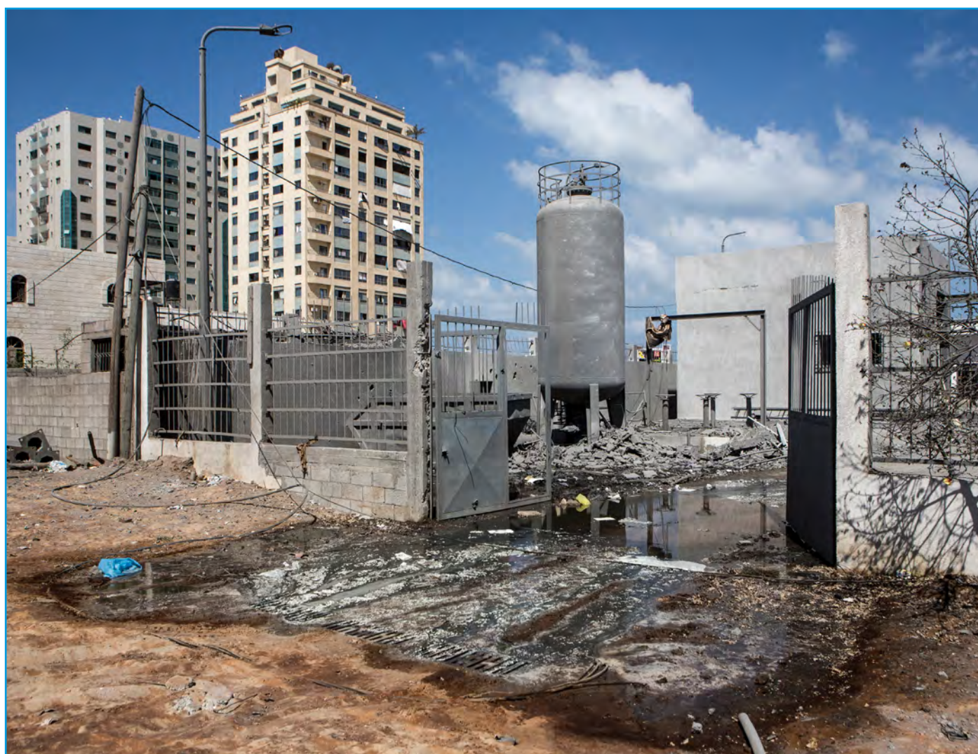
Gaza, South Remal waste water pumping station was damaged during bombings. Photo by Ann Paq @ ICRC
