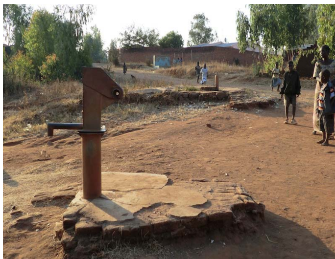
Figure 5: Derelict water point, Masitimale VDC, TA Kwataine, Ntcheu district (25 July 2012)
